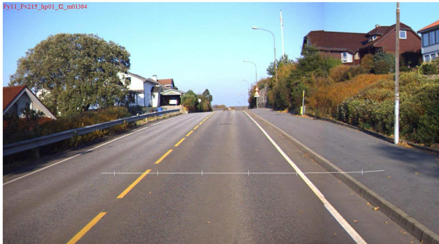
Fv 215 – Hp 1, km 0.020 – 1.720
